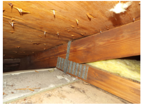
Toe - Nail - only 2 nails
