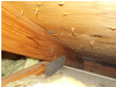
Toe - Nail - only 2 nails
